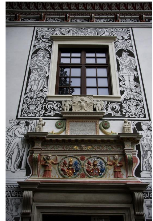
The wedding palace in Bytča - portal
